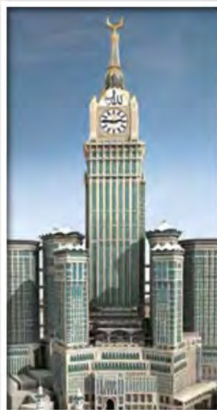
DOKAEE TOWER -H PLAZA - SAUDI ARABIA - 5mtrs
