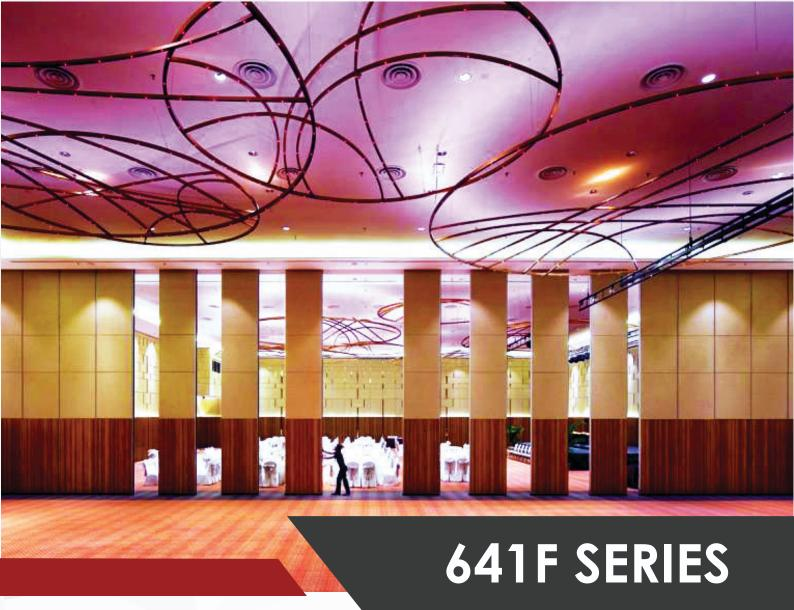
These rugged steel panels resist daily wear and tear and have a one-hour fire rating. They are an excellent choice for meeting rooms, heavy-use facilities, or wherever local codes require a fire rated partition.
